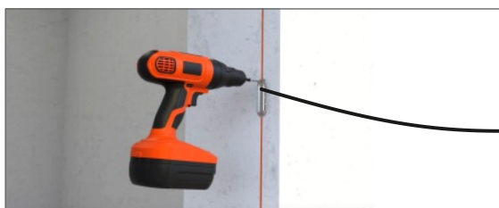
3 - Attach Clips to the Wall with suitable SS fasteners
