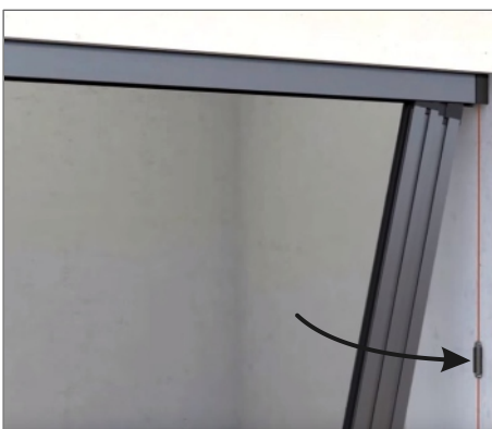
7 - Insert Mesh pack into the Top Guide. Then push Mesh Pack firmly onto the Clips. 'Clicks' If multiple doors insert the Train connector strip(s) first to join Doors together.
