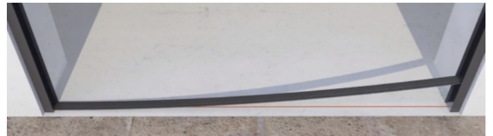
6 - After cleaning the floor area, attach Bottom Rail to the Floor with attached DS tape
