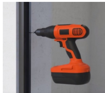
5 - Attach the U profile to Wall with suitable SS fasteners. (to ea side of Magnet)
