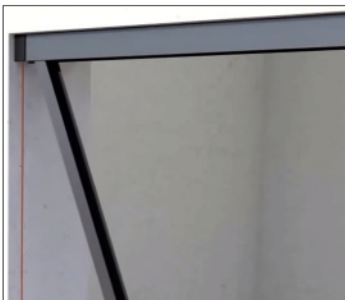
4 - Insert the U Profile (with Magnet) into the Top Guide
