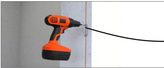
3 - Attach Clips to the Wall with suitable SS fasteners
