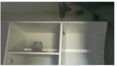
Working from one end... Clip on second vertical panel. Then insert Shelves or Rail between these two panels. Square up second panel, then secure suspension bracket in place. Then lock shelves (if any) between the first two panels.
