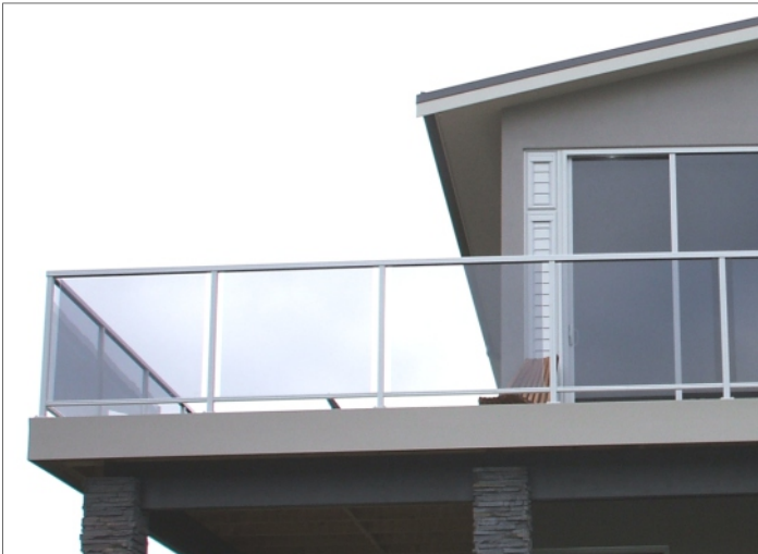
Juralco Viking® Balustrade showing Full Height glass with Handrail and Bottom Rail
