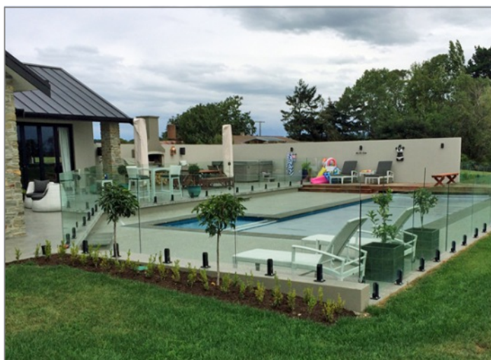
Juralco Edgetec Mini Post Framless Balustrade Top Fix to Tiled Concrete Deck. Pool
