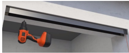
2 - Attach Top Guide to the Ceiling, with suitable SS fasteners. Pack if necessary; must be no greater than 10mm out of parallel to floor.
