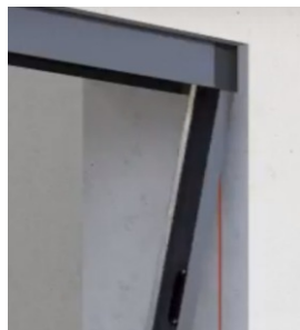
4 - Insert the U Profile (with attached clips) into the Top Guide
