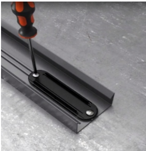
3 - Attach Clips to the U Profile (x 2 for Twin Door)
