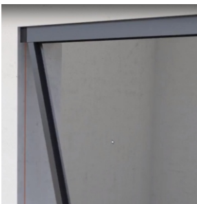
6 - Insert the other U Profile (with Magnet) into the Top Guide (for Twin doors this profile has clips)
