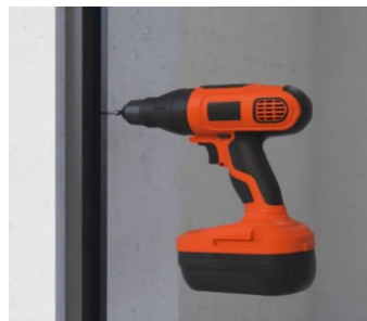
7 - Attach the U profile to Wall with suitable SS fasteners. (to ea side of Magnet). For Twin Doors as in 5 above
