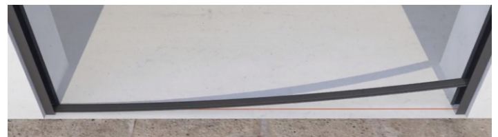
8 - After cleaning the floor area, attach Bottom Rail to the Floor with attached DS tape
