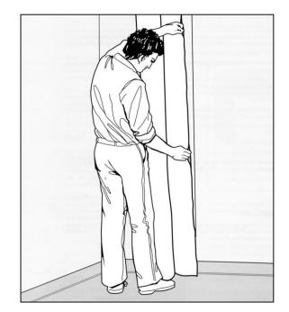
Back roll the wall material (face in) in the long direction. Place edge of wall material on plumb line and unroll into adhesive. Roll out the sheet little by little into the adhesive.
