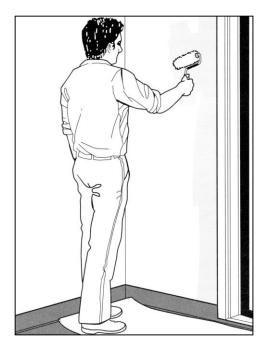
Apply adhesive on the wall area where the first sheet will be installed and a few inches past the seam edge. Apply adhesive in accordance with manufacturer's instructions. Use a 'lambs hair' roller. If you prefer to apply the adhesive with a fine-notched trowel, we recommend that you even out the adhesive over the surface with a roller-otherwise there is a risk that the trowel pattern in the adhesive will later show through the wall covering.
