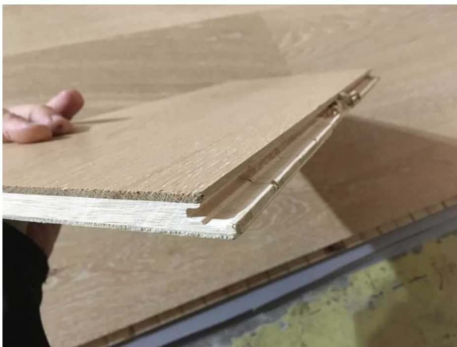
Figure 2: Section view of flooring
