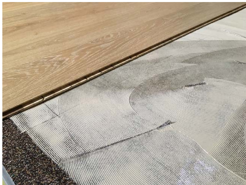
Figure 2: Applying Uzin adhesive to the Regupol 4515 underlay
