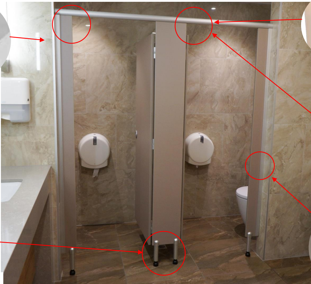
Anodised aluminium slimline headrail with snap headrail inserts
