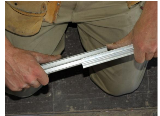
Slide starter bar top section over support bar
