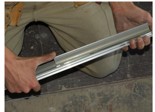
Use starter bar bottom section to ensure position is correct
