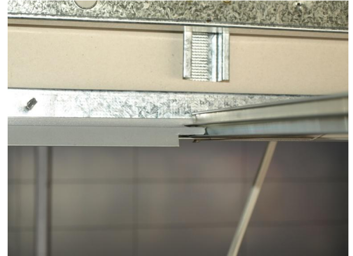
This can be achieved by using a spacer cut to the appropriate width
