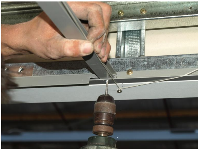
Once in position drill through angle and support bar.
