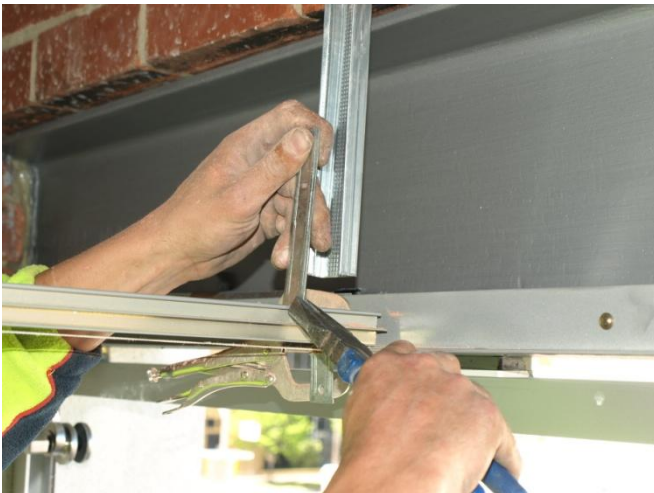
Be sure to close the bottom leg of support clip
