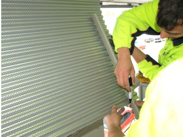
Mark sheet to be cut using a whiteboard marker.
