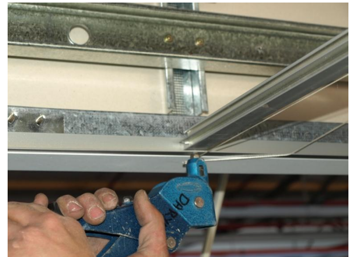
Then fix in position using a pop-rivet
