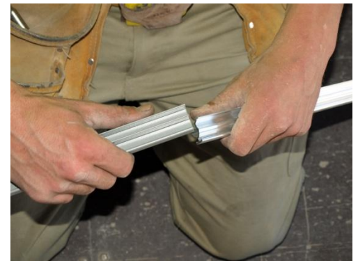
Align top of support bar and starter bar top section
