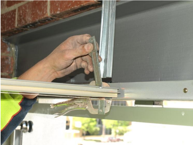
Support clip is attached to fastrack support bar
