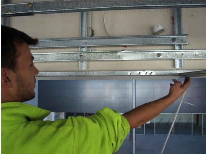
Prepare to fix Support bar to angle by ensuring the correct gap has been allowed
