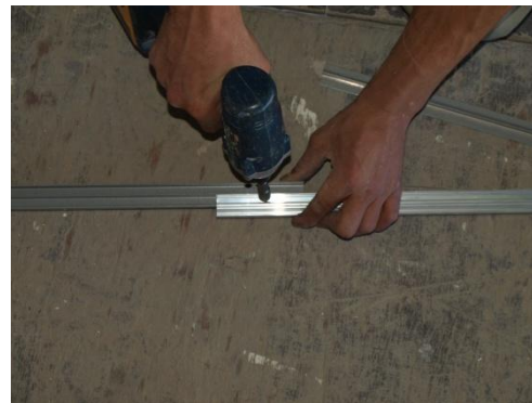
Fix top section to support bar using a self drilling screw
