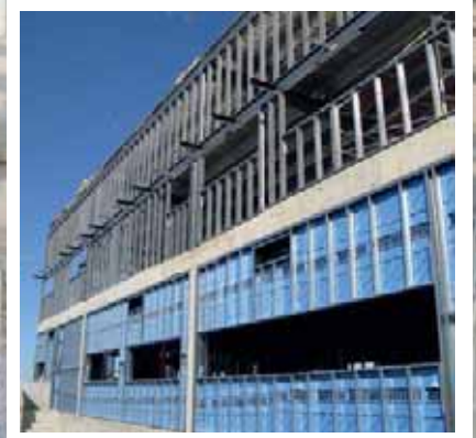
External Infill Framing Between concrete and steel structures
