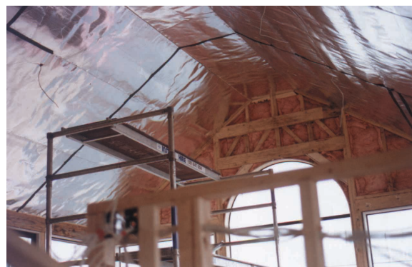
dBX is used in roof applications for the control of internal and external environmental noise problems.
