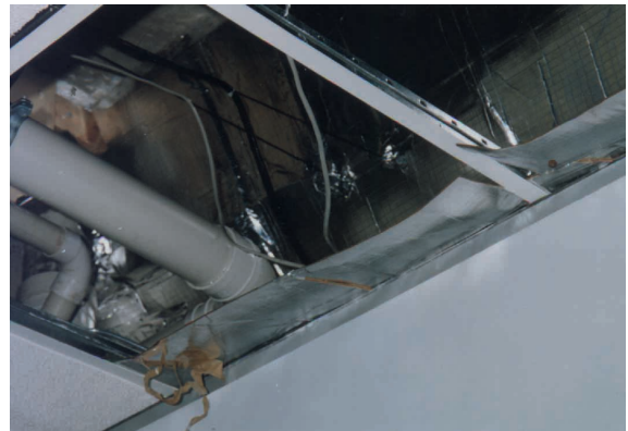
dBX is easily joined and penetrations resealed. As a non PVC product, taping and sealing penetrations is possible with a tape system.
