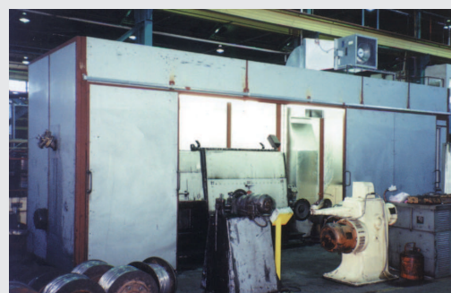
Large localised enclosure constructed in-situ in cable making factory
