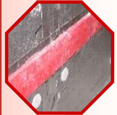
VFB Plus Ventilated Fire Barrier Installed between Insulation Panels
