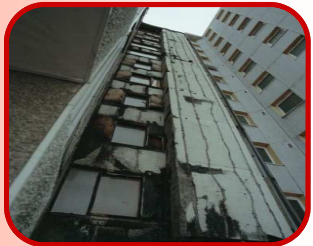
Evidence of Rapid Fire Spread behind a cladding
