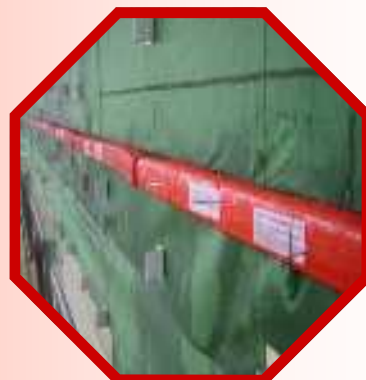
FF109/125 Ventilated Fire Barrier Installed prior to cladding panels
