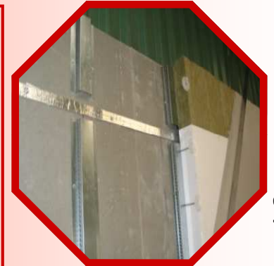
FF102/25 Ventilated Fire Barrier Installed behind cladding system
