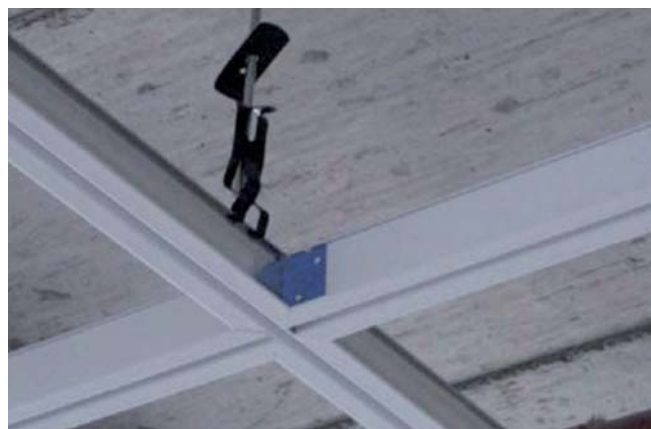
Clean mitred cross runner intersection.
