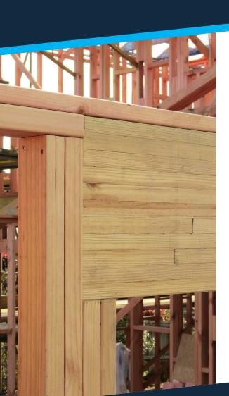
Hyne Beam 15 is the perfect choice for long spanning beams.and lintels. Glulam offers a number of benefits over other engineered alternatives such as:
