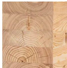
Example of end checking contained within lamination of Glulam
