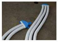
The round shape of the ducts and valve collectors.
