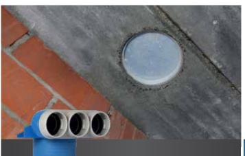
The sealing caps and lids provided with the ducts, distributors and valve collectors ensure that no building materials and debris can come in the pipes and components during the installation.
