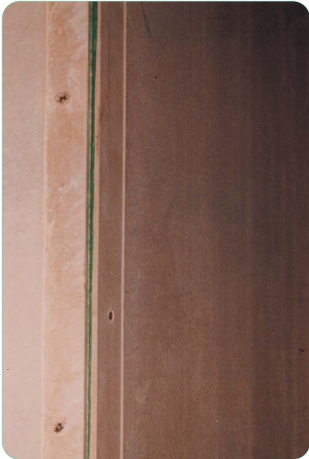
FIGURE 34 External corner with reinforcing mesh stopping
