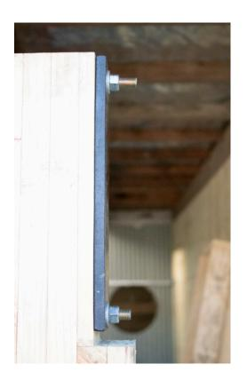
5. Stand the entire portal into place, level, brace and tighten the hold down bolts using 50x50x3mm washers.
