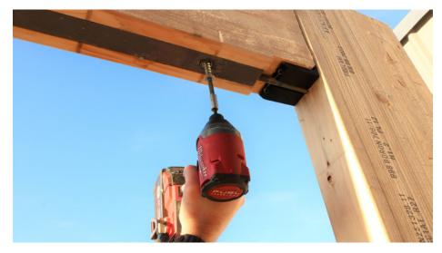
12.Install backing plate with curve facing out, install Belleville washers (cone facing out) and tighten to 50Nm torque to flatten both the Belleville washer and the plate against the timber leg.
