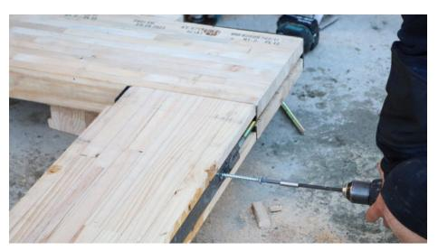
4. Tighten the M12 bolts to 50Nm Torque and flatten the Belleville washer and 12mm backing plate flat against the portal leg.
