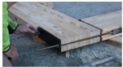
3. Screw the top and bottom arrow head connectors into the PLX20 beam using VGS 9x160 screws.
