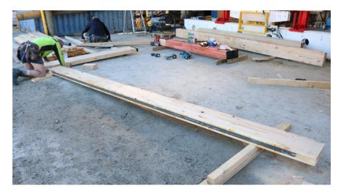
2. In both portal legs, install the bottom M12 threaded rod assembly, through the 12mm backing plate (curved ends facing out) and using the Belleville washers between the nut and 12mm backing plate, and nail the L bracket on the beam side of the column into place.
