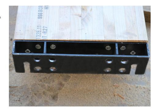
5. Install the hold down thru bolts for concrete, or M12 threaded rods for timber sub floors.
