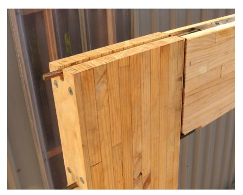
10. Screw the top and bottom arrow head connectors into the PLX20 lintel using VGS 9x160 screws.
