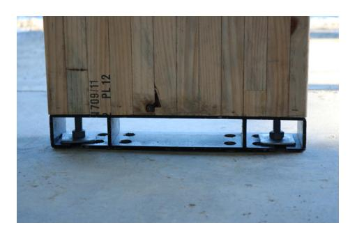
7. In both portal legs, install the bottom M12 threaded rod assembly, through the 12mm backing plate (curved ends facing out) and using the Belleville washers between the nut and 12mm backing plate, and nail the L bracket on the lintel side of the portal leg into place.
