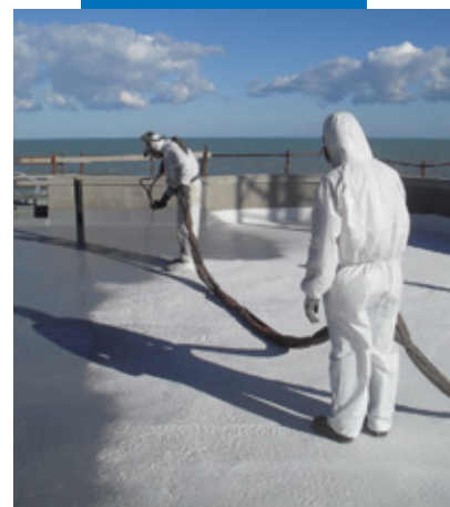
Application of Purtop 400 M over Triblock P
