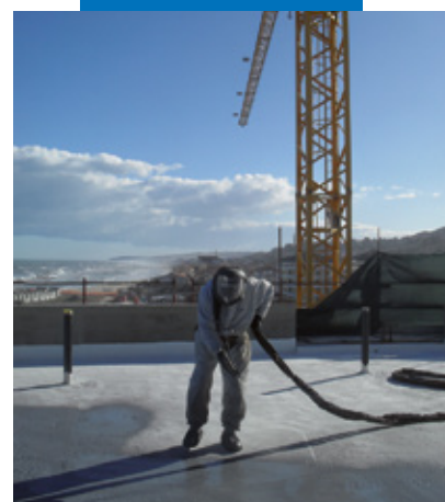
Application of Purtop 400 M over Triblock P
