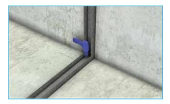
Then use the fixings to secure the C-track.
