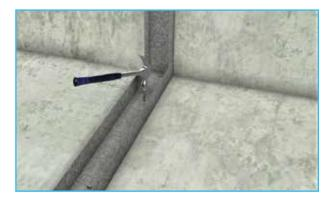
If the surrounding surface is uneven or if you're not sure you have a good seal, add a continuous bead of fire-rated sealant around the perimeter of the C-track where it contacts the surrounding surface.
