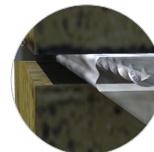
Installs into the mortar joint to provide an **inconspicuous repair** and preserve the appearance of the structure
