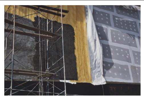
**Waterproof membrane.** This membrane should be applied after the installation of the boards to protect them from the permanent contact of the humidity on the façade and prior to the cladding components.
