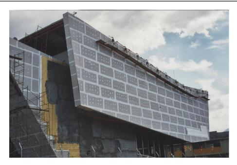
**Humidity protection.** Vapour permeable membrane is recommended as a layer between the metal frame and the boards installation to control the excessive humidity driven by the exterior pressure and the wind loads. In any case the back surface should always be protected against excessive water absorption to maintain the boards mechanically stable.
