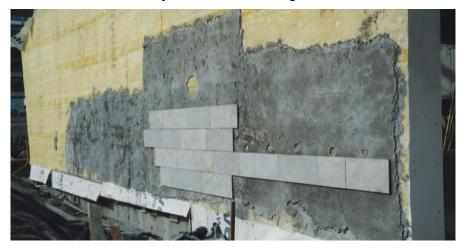
**Watertightness of the façade system.** Whatever the cladding application, special attention should be given to the water management on the façade solution. ETERPAN® MD backerboard should be protected against the permanent humidity on the exposed surface but also on the unexposed side where any risk of condensation or ponded water should be avoided.
