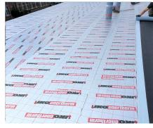
IKO Enertherm ALU is used for the insulation of flat roofs for new construction or refurbishment projects on concrete, steel deck or timber substrate.
