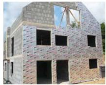
IKO enertherm is used for the thermal insulation of cavity walls.
