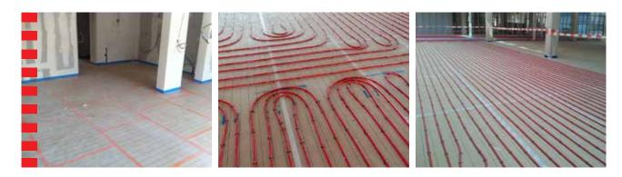
IKO enertherm is used for the thermal insulation of floors.
