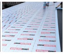
IKO Enertherm ALU TAP is used for the tapered insulation of flat roofs for new construction or refurbishment projects.
