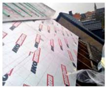
IKO enertherm is used for the thermal insulation of pitched roofs.
