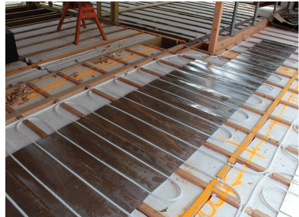
Spreader plate installation for upper floors or elevated ground floors
