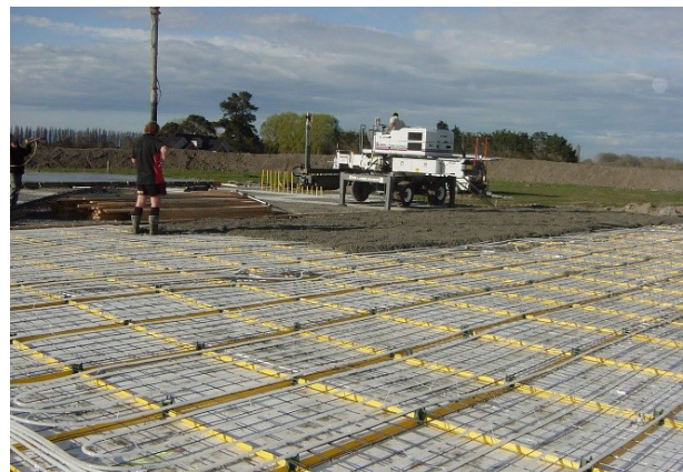
Method 2: Installation using crack inducement.
