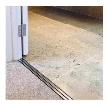
The JESANI® Door Channel is the new innovative linear channel floor waste drain to supersede all other floor wastes.
