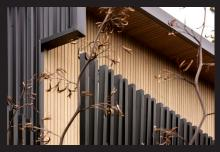
No. of coats exterior new work: 2 coat initial system 1st coat factory applied or site applied prior to fixing. 2nd coat 30-90 days after fixing.
