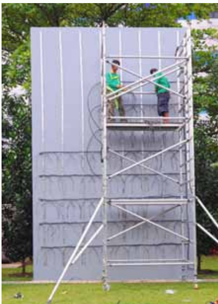
Installation of VGM®
