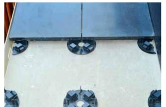
VersiPave® separated into halves to enable flush placement along edges.
