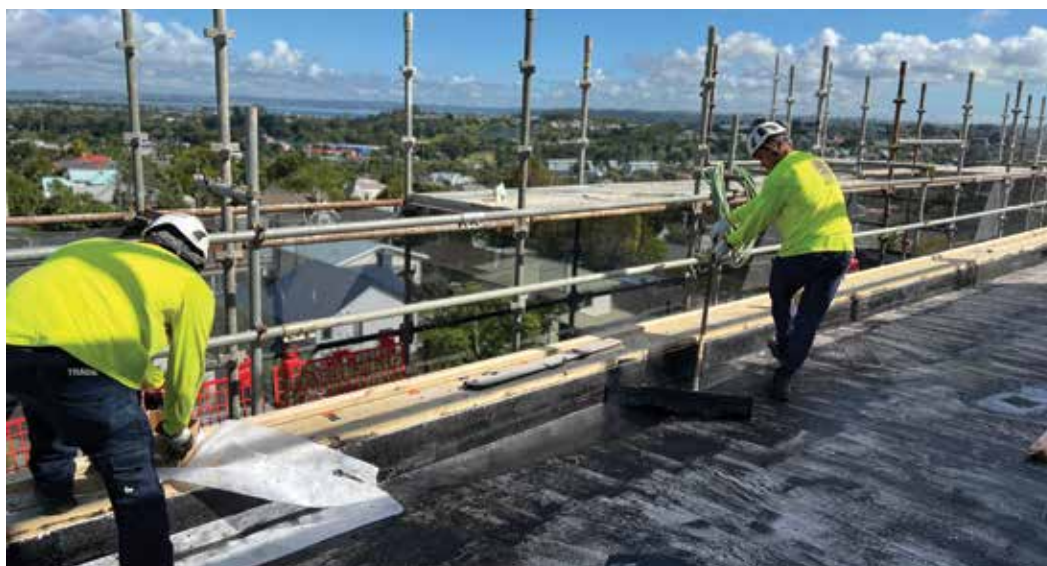
Hydrotech MM6125® system Installation in progress.
