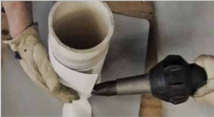
STEP 2. Tack weld PF340 to fit penetration
