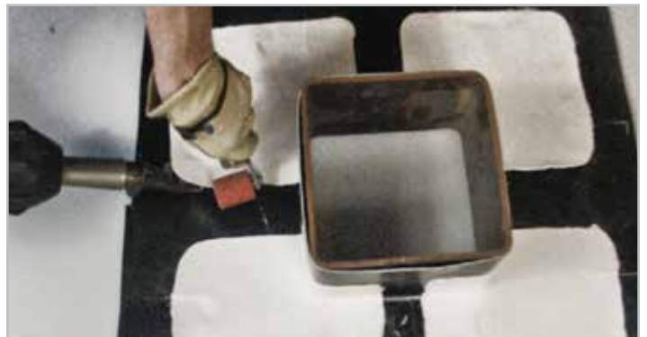
STEP 6. Install at all four corners
