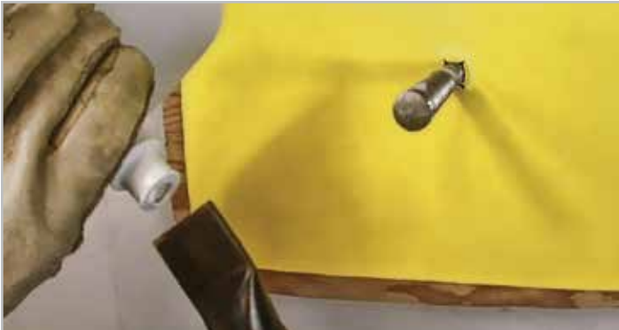
STEP 4A. Heat trimmed PF-150 cut end
