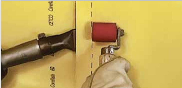
STEP 2. Pre Weld Placement
