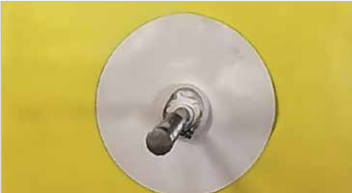
STEP 8. Tightly secure hose clamp
