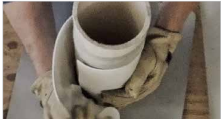
STEP 1. Place PF340 around penetration
