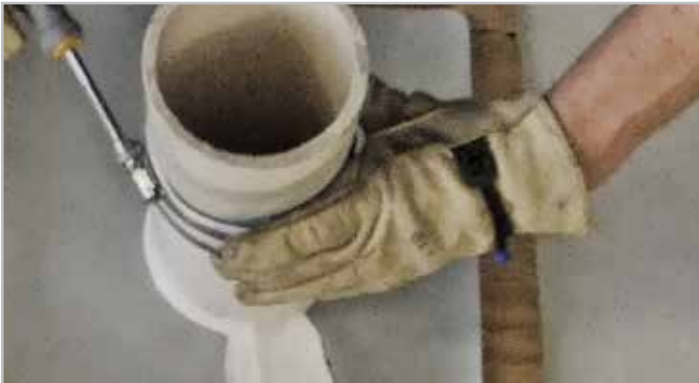
STEP 7. Install second hose clamp
