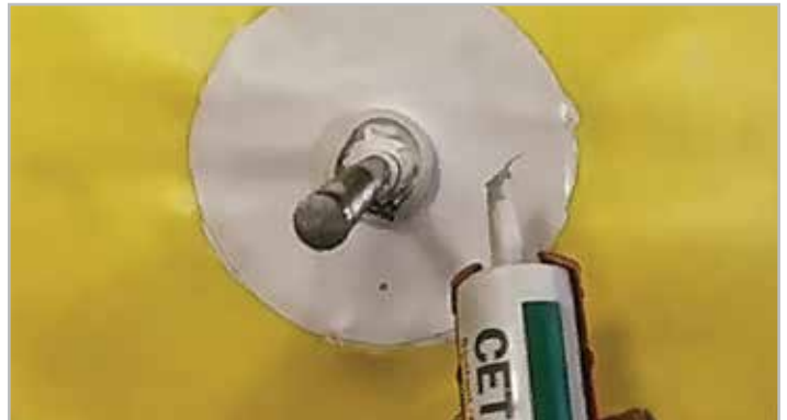
STEP 10. Apply CETSEAL at termination
