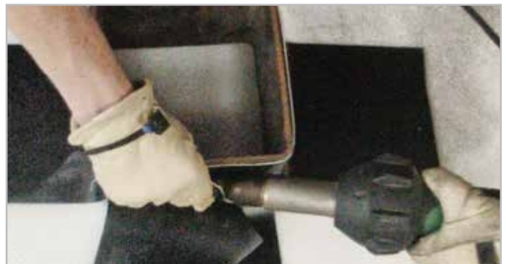
STEP 2. Target flashing tack weld
