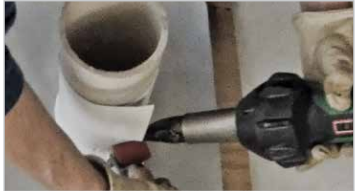
STEP 4. Weld vertical overlap seam up stack
