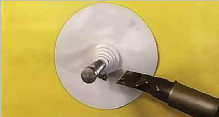
STEP 7. Hot-air applied to stepped stack
