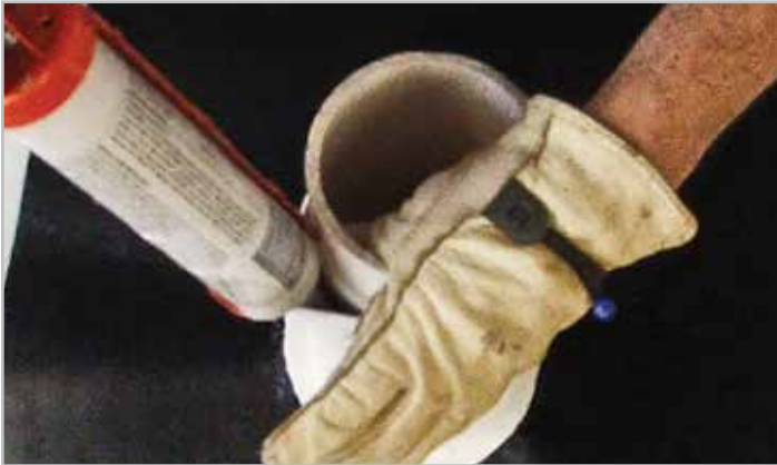
STEP 7. Install AKWASWELL bead
