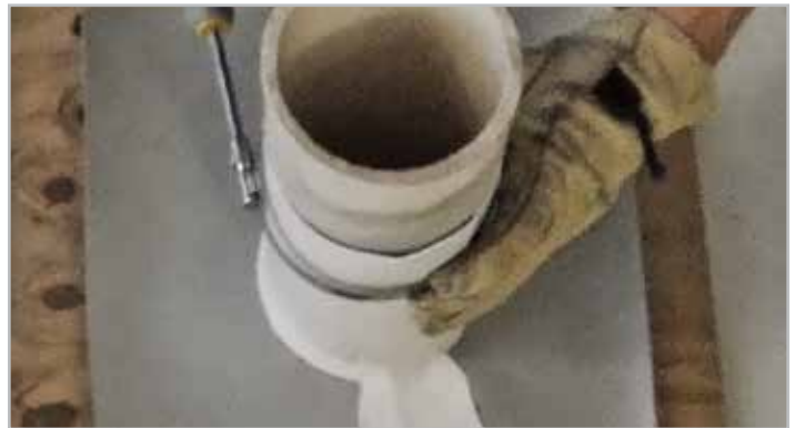
STEP 5. Install lower clamp
