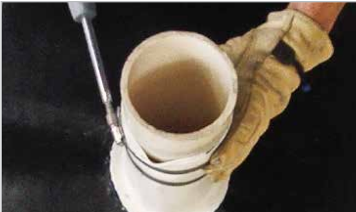
STEP 8. Install second clamp
