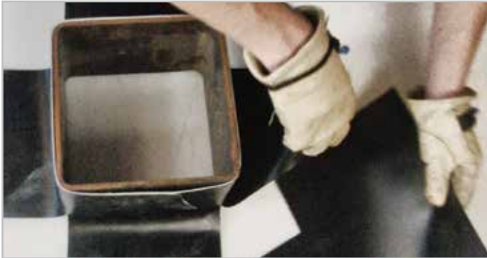
STEP 3. Place corner target patch
