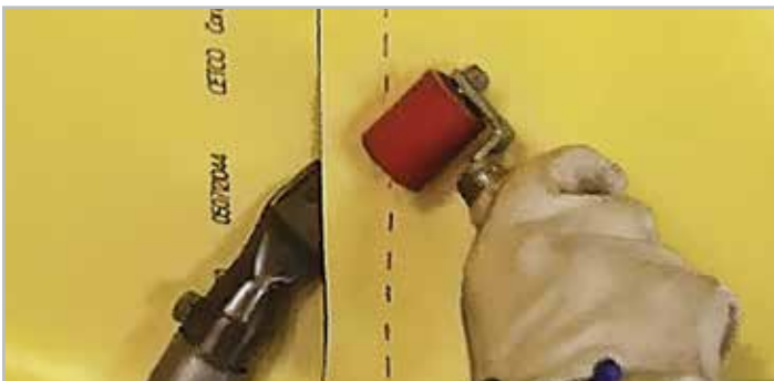
STEP 3. Final Weld Placement
