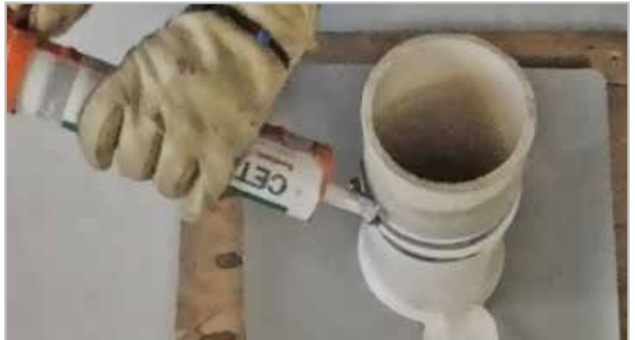
STEP 9. Apply CETSEAL bead at termination
