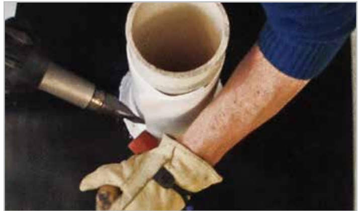
STEP 5. Weld Vertical NR to target piece
