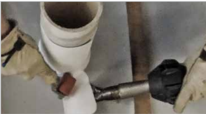
STEP 3. Weld PF340 overlap at base flange
