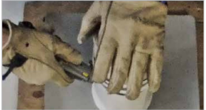
STEP 8. Trim excess membrane flush with top edge of clamp
