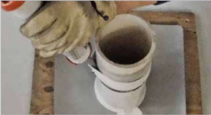
STEP 6. Install AKWASWELL bead
