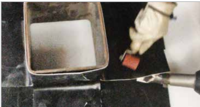
STEP 4. Weld target patch in place
