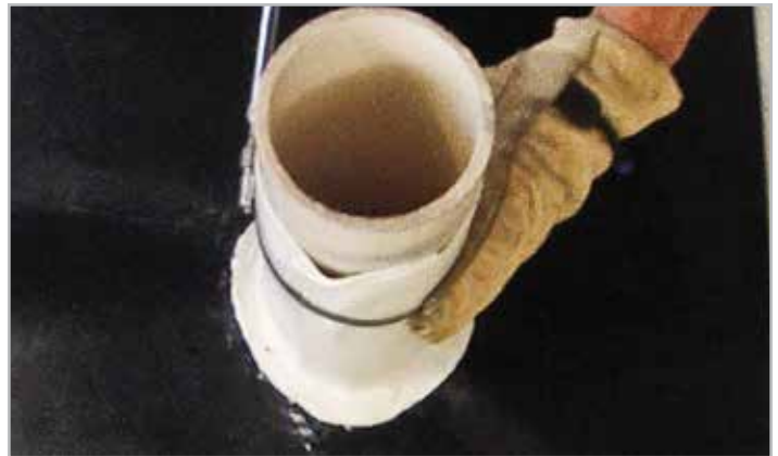
STEP 6. Install lower clamp
