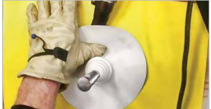
STEP 5. Tack weld PF-150 flange
