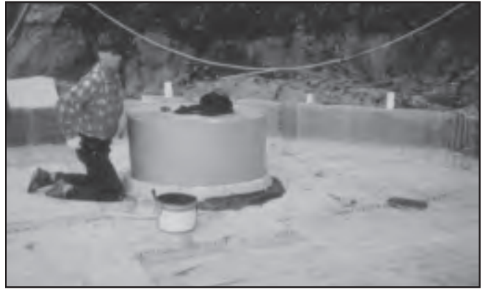
Figure 1.16 - Cut Voltex to closely contour penetrations.
