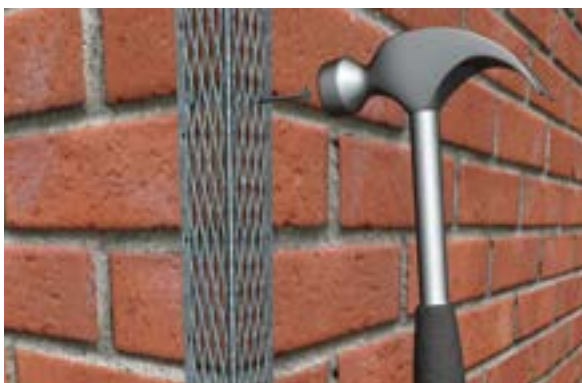
■ NAILING INTO THE MORTAR ON MASONRY WALLS
