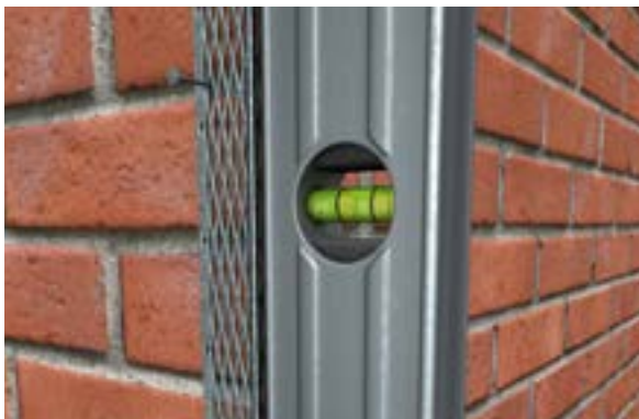
■ ENSURING THE BEAD IS PLUMB AND STRAIGHT
