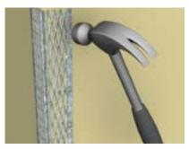
Beads can be attached by nails or a staple gun at not more than 500mm centres down the legs of the bead, and not more than 100mm from each end.
