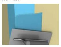
Apply second coat to a width of approximately 120mm. Allow to dry, then remove any excess and lightly sand if necessary.
