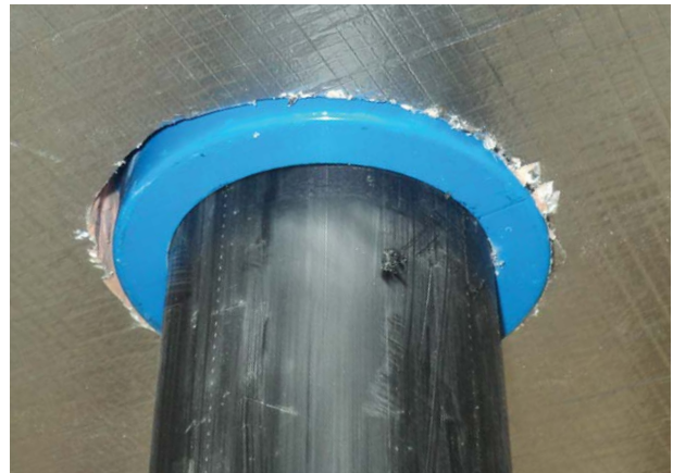
Figure 6. Penetration example - Kooltherm K10 G2W Soffit Board installed tight around the fire collar and HDPE service pipe.
