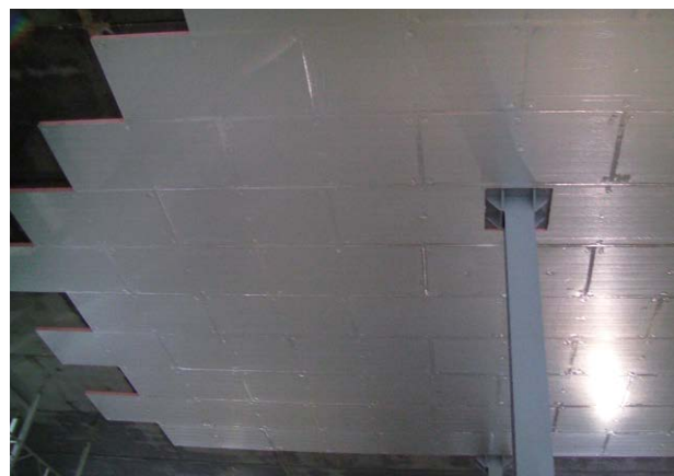
Figure 4. Board joints staggered.
