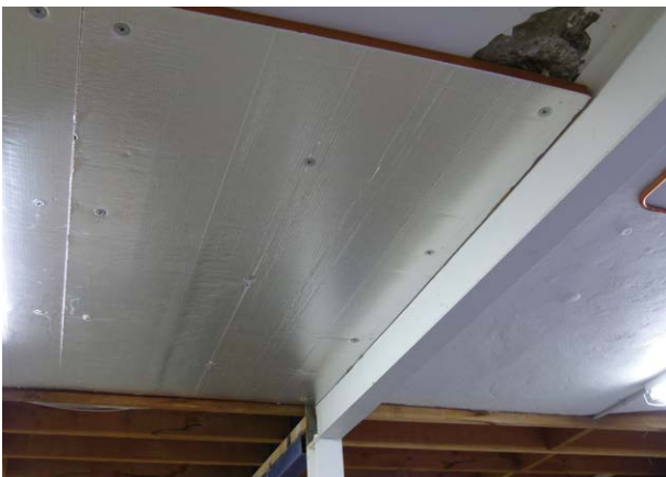
Figure 6. Penetration example - Kooltherm K10 G2W Soffit Board installed tight around the fire collar and HDPE service pipe.
