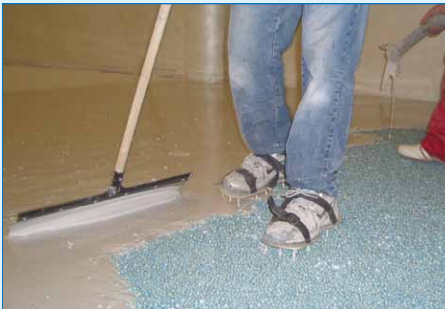
Application of Ultratop on the hardened surface of Dynastone Color
