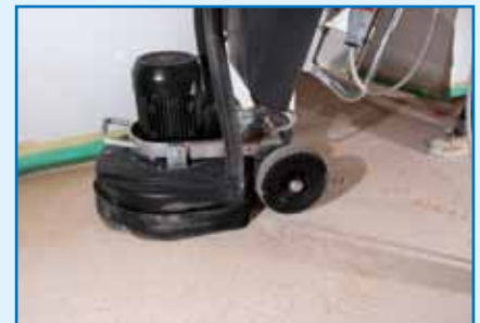
Dry polishing the flooring
