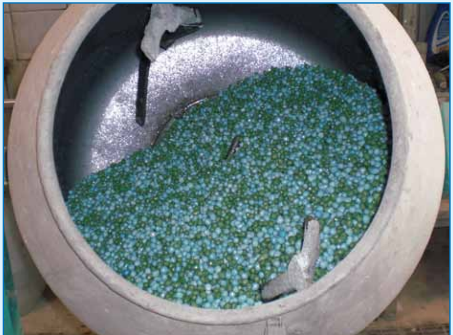
Preparing the mix of Dynastone Color + Mapefloor I 910
