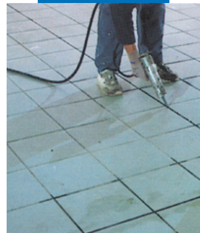
Sealing ceramic tile floor with Mapesil AC
