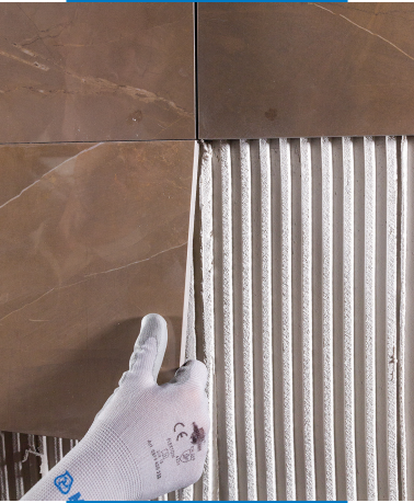
Installation of ceramic wall tiles
