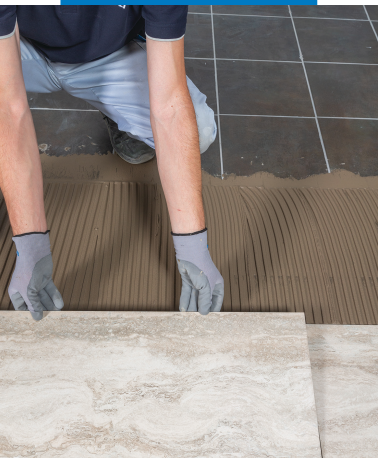
Installation of stone-effect floor tiles over existing flooring
