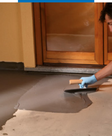
Waterproofing of terraces by trowel
