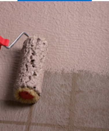
Waterproofing of details by roller
