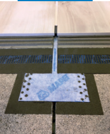
Mapeband Easy applied around a control joint in the screed
