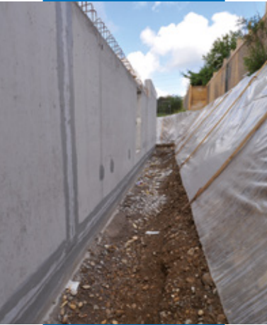
Sealing structural joints in retaining walls
