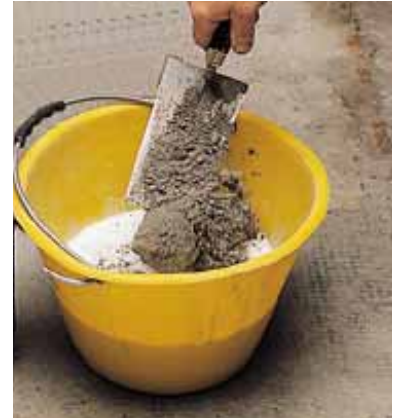
Mixing Mapecem with Planicrete to make an anchoring slurry
