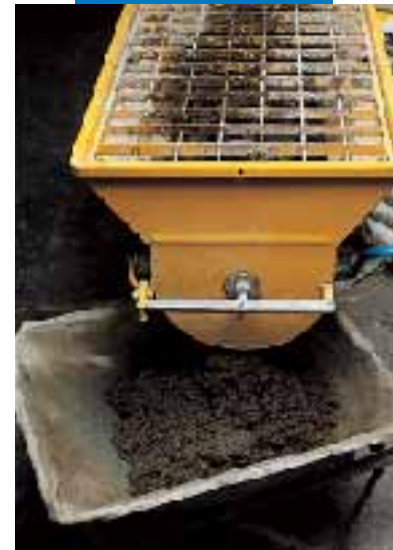
Mixing Mapecem in a mini-batcher
