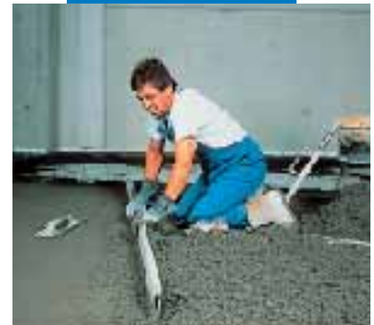
Using the straight-edge
