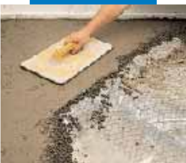
Covering pipes with Mapecem and reinforcement netting
