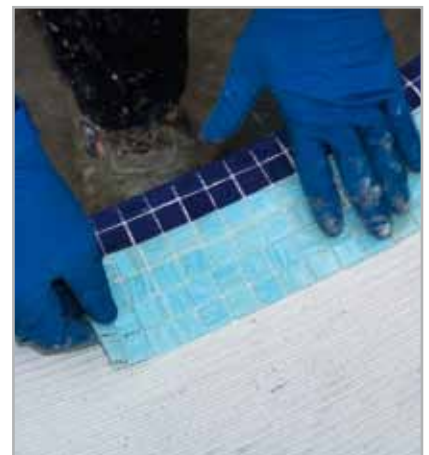
Fig. 5.4 - Installing a mosaic lining
