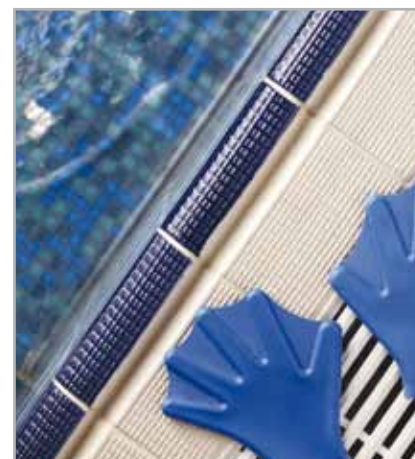
Fig. 5.5 - Grouting the lining with ULTRACOLOR PLUS
