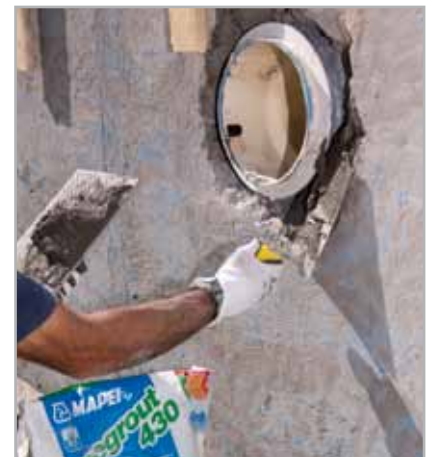
Fig. 4.3 - Reintegrating a substrate with MAPEGROUT 430
