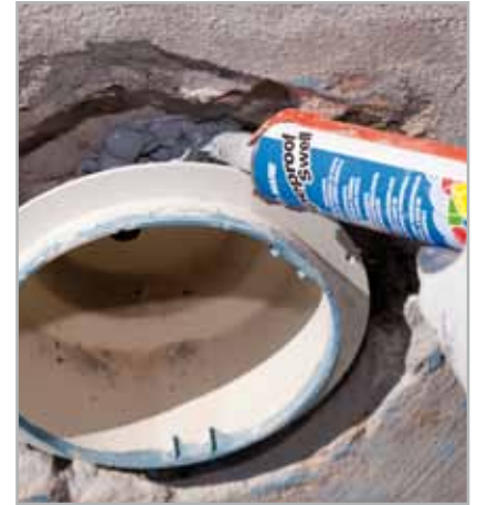
Fig. 4.2 - Forming a seal with MAPEPROOF SWELL
