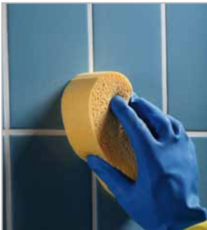
Fig. 5.8 - Final cleaning operation with a clean sponge
