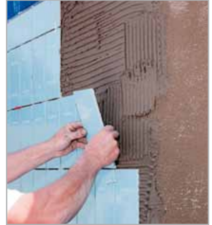
Fig. 5.2 - Bonding tiles to a wall with KERABOND mixed with ISOLASTIC
