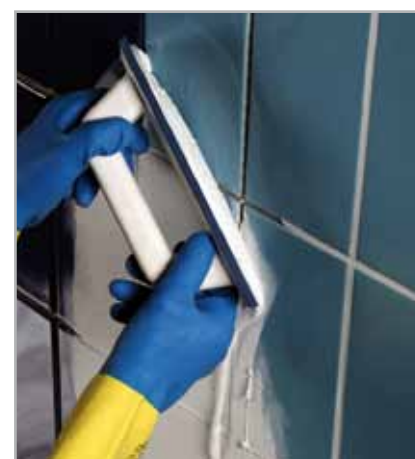
Fig. 5.6 - Grouting the lining with KERAPOXY CQ
