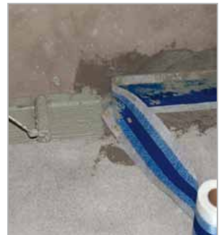
Fig 3.8 - Sealing and waterproofing fillets between a horizontal and vertical surface with MAPEBAND
