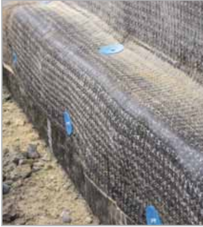
Fig. 3.3 - Waterproofing treatment along the base of the structure
