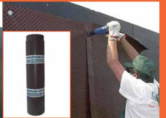
**10** - Fasten the bituminous membrane to the wall using the appropriate mechanical fastening systems at the overlapping points.
