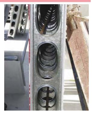
These holes are covered with a temporary patch (duct tape is often sufficient) until after pour. Later when the corners have a bead fitted and are flushed, these holes are patched and flush set.
