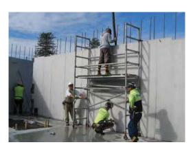
Consideration should also be given to the positioning of braces to provide the best results and also to minimise restriction of free movement by personnel around the site. If the walls are going to need to be filled off a mobile scaffold, it is preferable to run the braces in a way that leaves one face of each wall clear.
