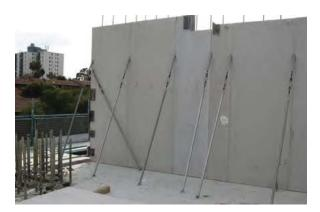
positions to push/pull the panel into alignment. AFS Logicwall® needs to be installed to achieve a tolerance of +/- 4mm over any 1800mm plane. In the case of corners it is not uncommon to use 3 or 4 braces.
