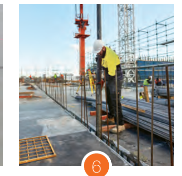
Core filled via a boom pump sees walls become load bearing
