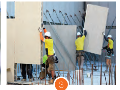
Lightweight panels can be readily positioned without craneage
