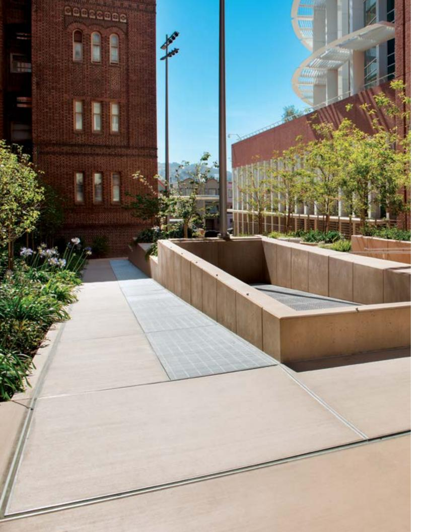
One of the largest base isolated hospitals constructed in the United States—able to glide 30 inches in every direction during a seismic event
